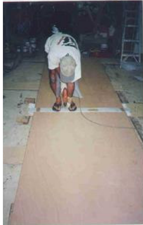
^ Standing on aluminium plate to drill holes.
