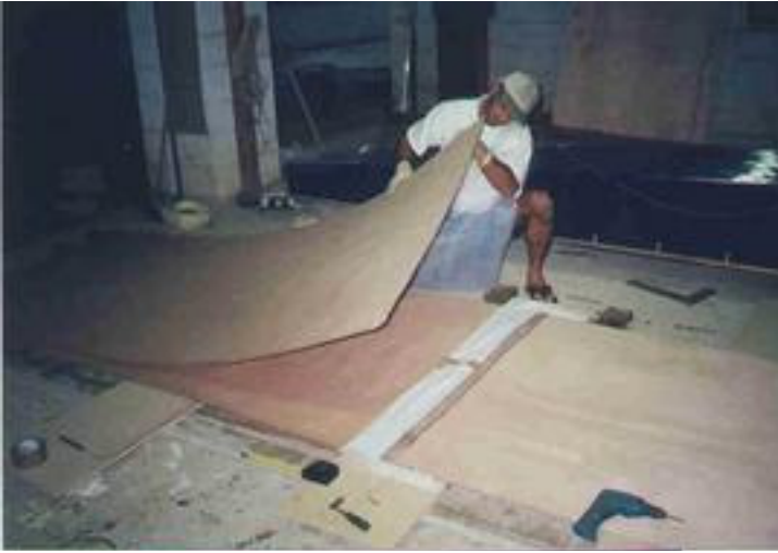
^ Separate ply with plastic - clamp joints for 24hrs.
