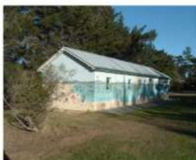
Iluka Iluka is used for activities
